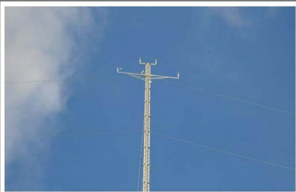
Photo 1: Close-up of mast top towards East
