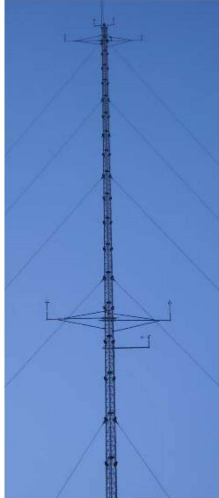
Photo 3: Mast measurement levels 54/57 m and 97/100 m
